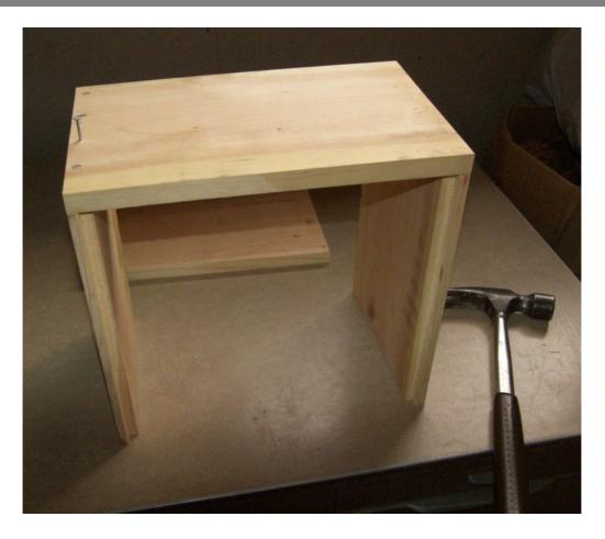
Flip the box assembly over and lay the other long side over the top of the two short sides. Fasten it in place. Congratulations on completing the main hive box assembly! Next we will add the top bars.
